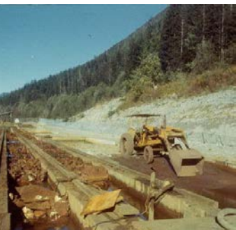
The Mount Sheer Townsite Launderers in operation
