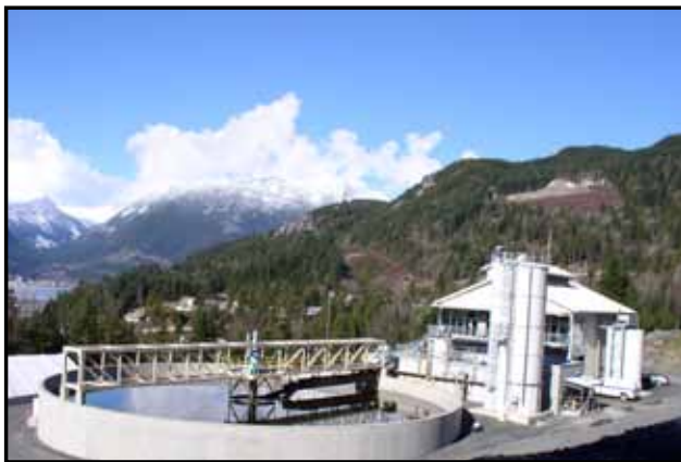
EPCOR Britannia Mine Water Treatment Plant
